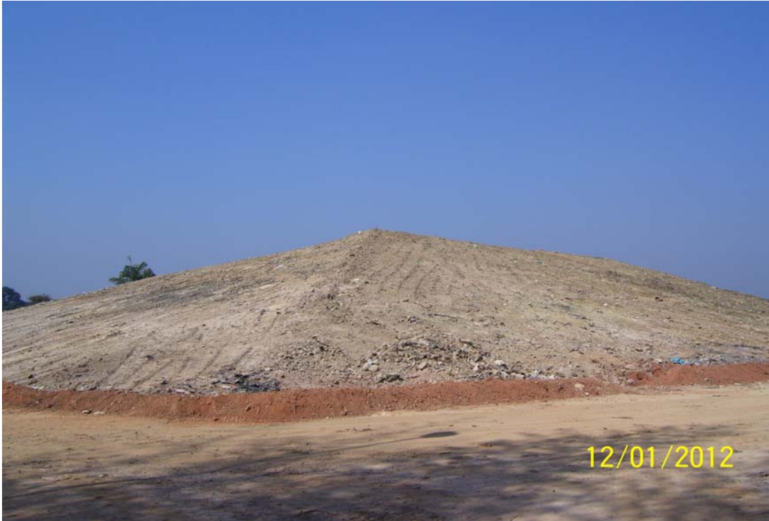
Figure 5.4 : Cell 1 before capping
