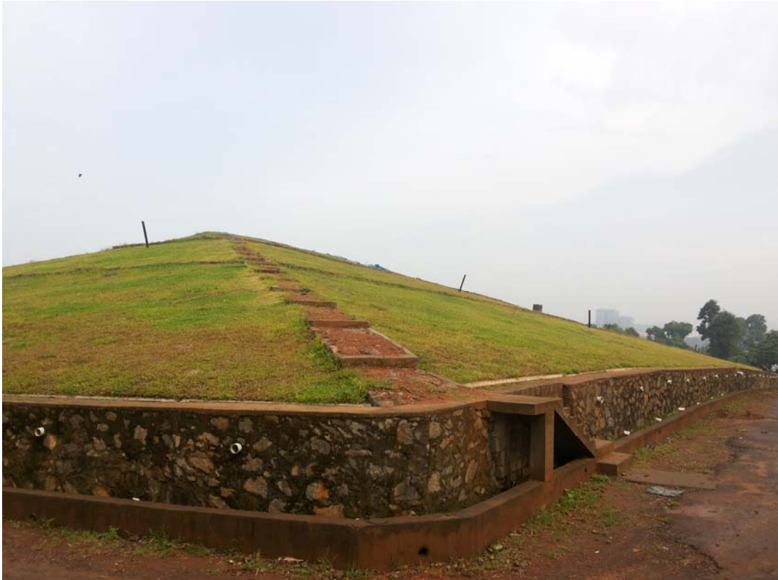
Figure 5.6 : Cell 1 after capping
