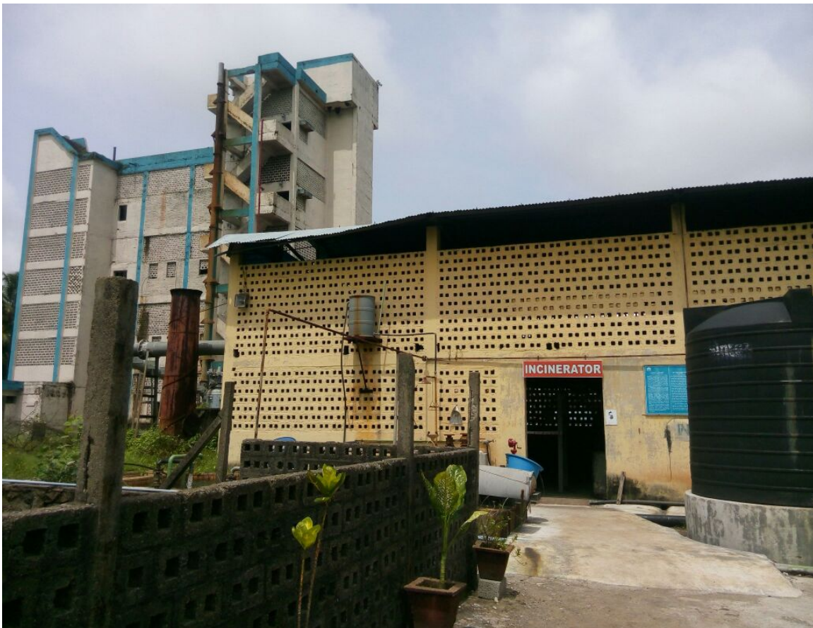
Figure 4.2: Hazardous Waste Incinerator at Hindustan Insecticides Limited (HIL)
